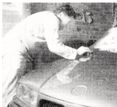
'Color' or 'Wet' sanding, if properly done, will result in a high-gloss, glass-like appearance.
