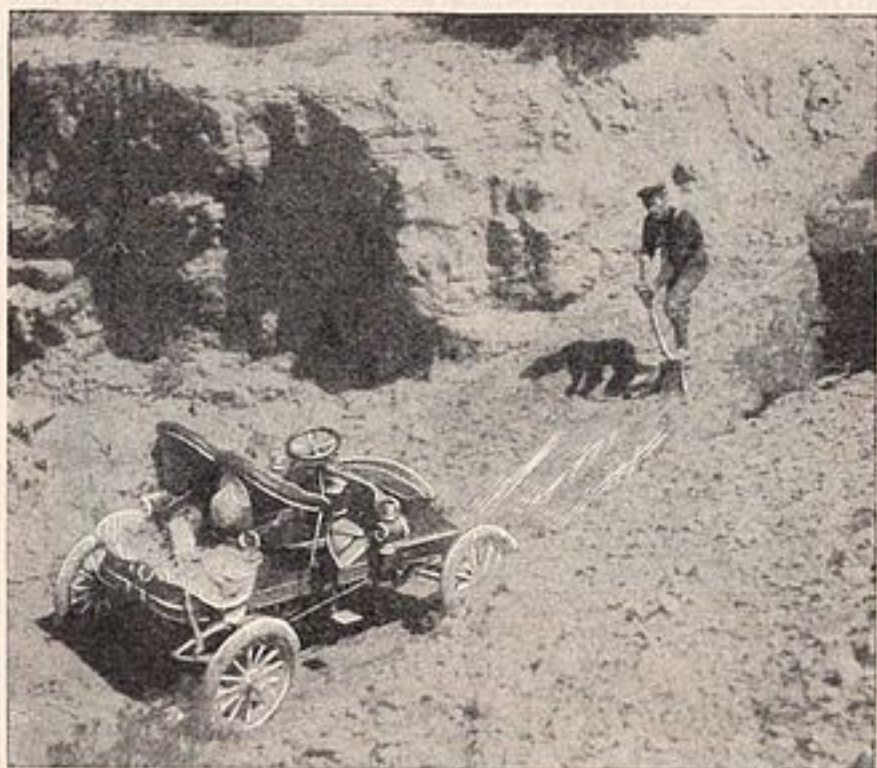
Fixing a bad spot in a road out of a canon near Point of Rocks, Wyoming
